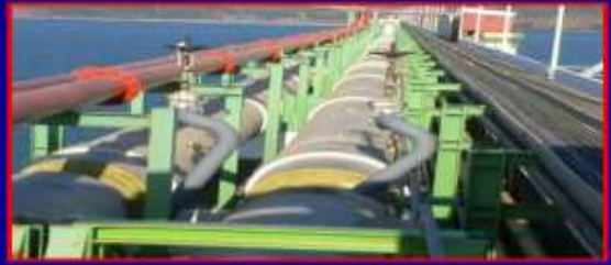
Ring Main Re-circulation Line Hook-Up
