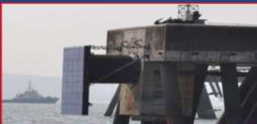
New Fendering System
