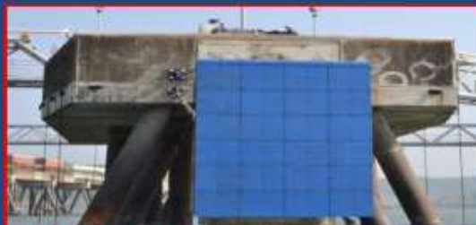
New Fendering System
